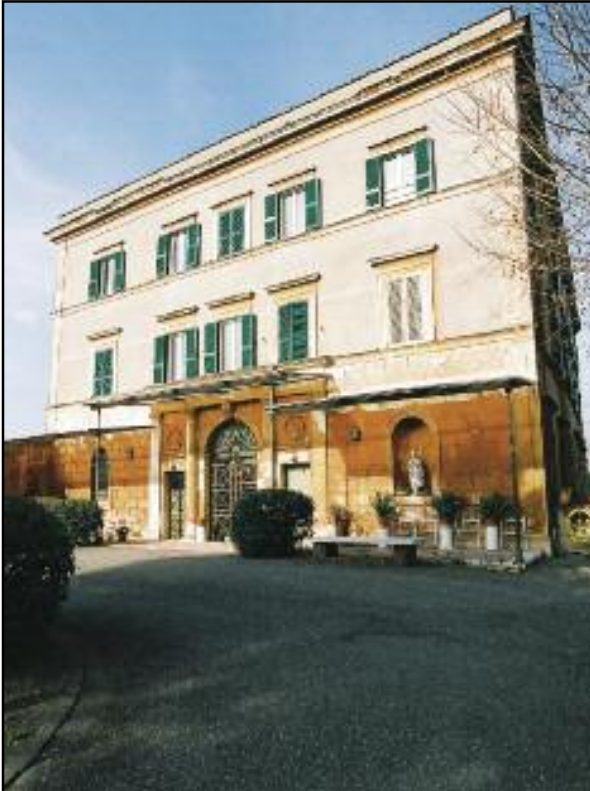
The Casa O'Toole as it looked before the renovations.
